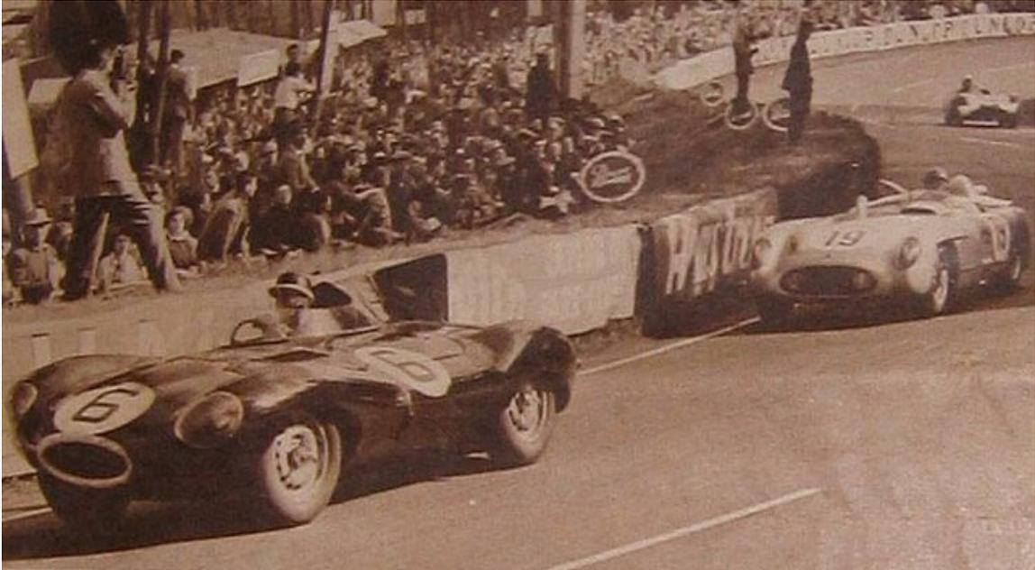
Jaguar entered the 1955 Le Mans 24-hour race with a version of the D-Type which has a bonnet seven inches longer than the standard model. Hence the name "Long nose D-Type". The car had a cover above the passenger space, a fin behind the driver's head and a higher windscreen.
